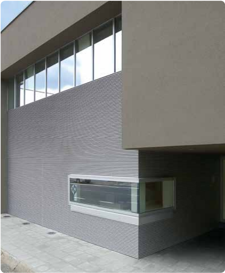
Ref. Private House/office – Menden (B), Arch. Philippe Guilbert
